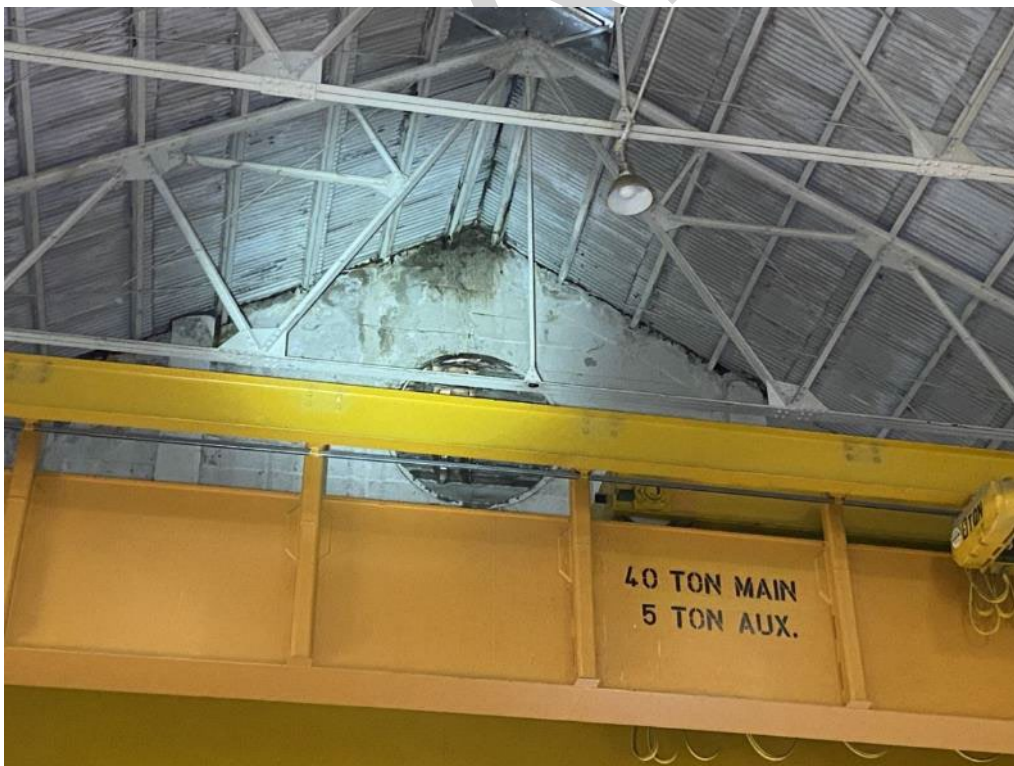
Figure 3.6-12. Staining under Roof at Main Entrance to the Powerhouse
