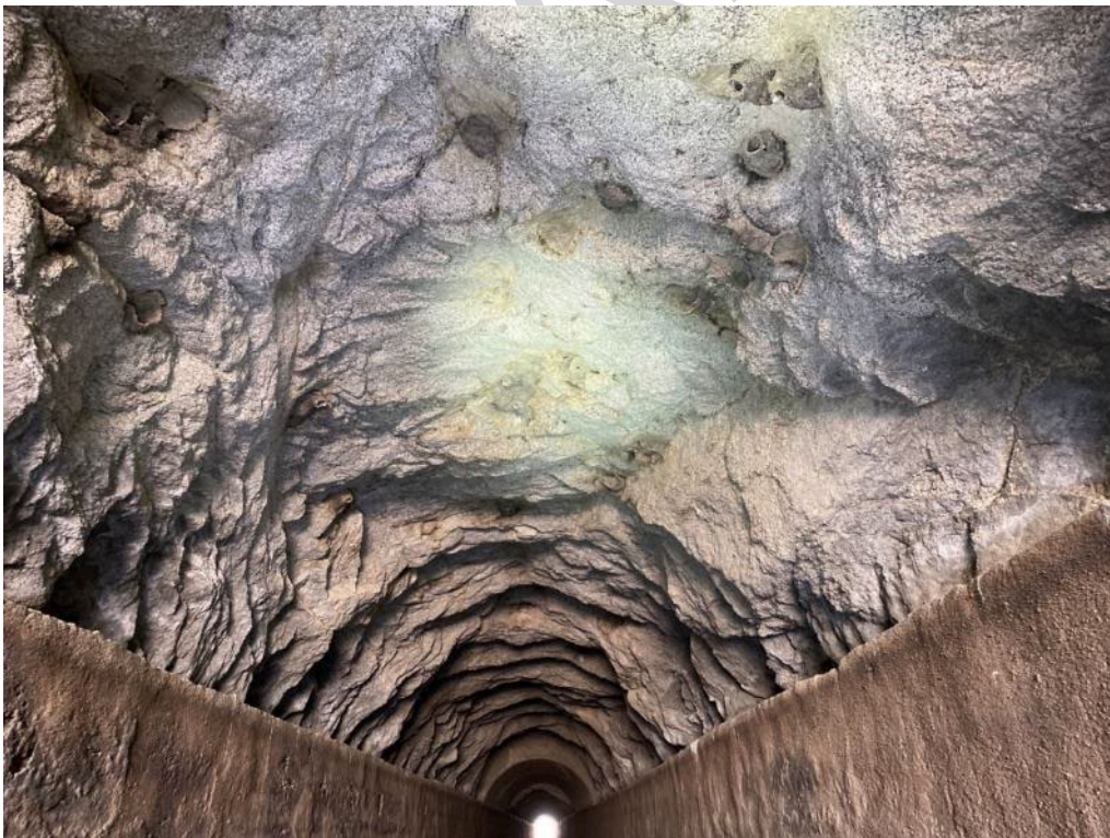
Figure 3.6-10. Granite Ceiling of Tunnel No. 2
